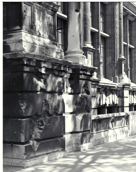
Photograph of the Aston Webb facade of the V&A Museum. Exhibition Road. Bomb damage during World War 2. V&A Archive, MA/32/123, neg. 41656
