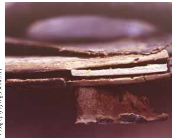
Figure 3. Fillets of balsa wood inserted between the boards
