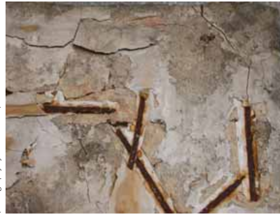
Figure 4. Tile back: detail of iron dowels (2043-1899)
