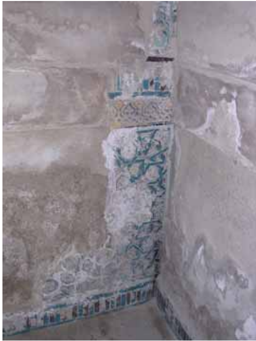
Figure 2. White efflorescence on damp (previously tiled) walls indicating the potential for soluble salt migration
