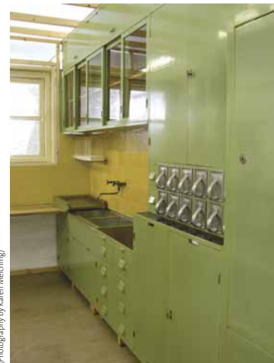
Figure 3: Kitchen surfaces repainted in the original green colour
