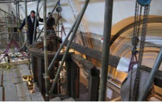
Figure 2b. Bressummer beam removal
