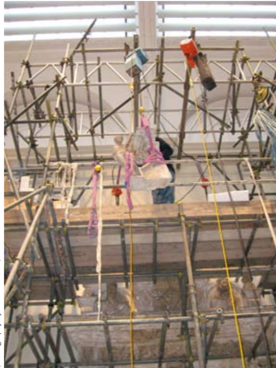
Figure 7. Installation of the dormer window, raising stone figure into position
