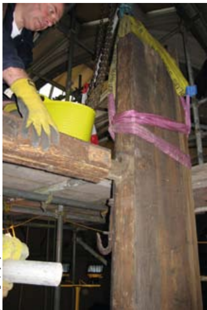
Figure 3a. Vertical timber being removed
