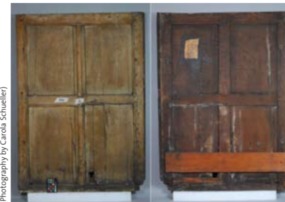
Figure 1 (a & b). Front and back of interior panel No. 39 with losses at the lower horizontal rail and lower corner joints with the softwood repair screwed to back
