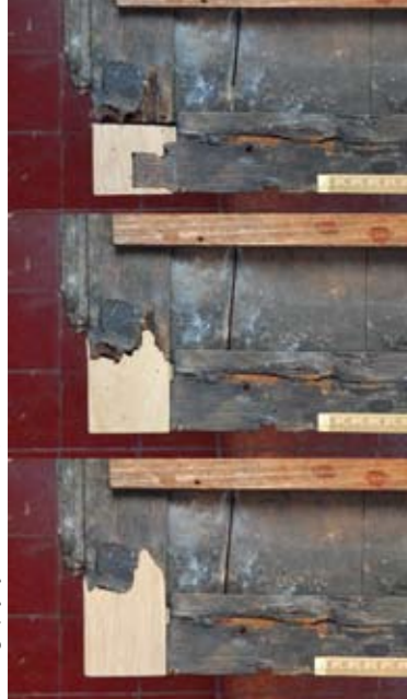
Figure 2. Layered loss compensation at the proper left lower frame joint at an interior panelling
