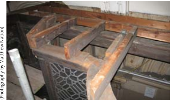
Figure 1a. Roof boards after removal
